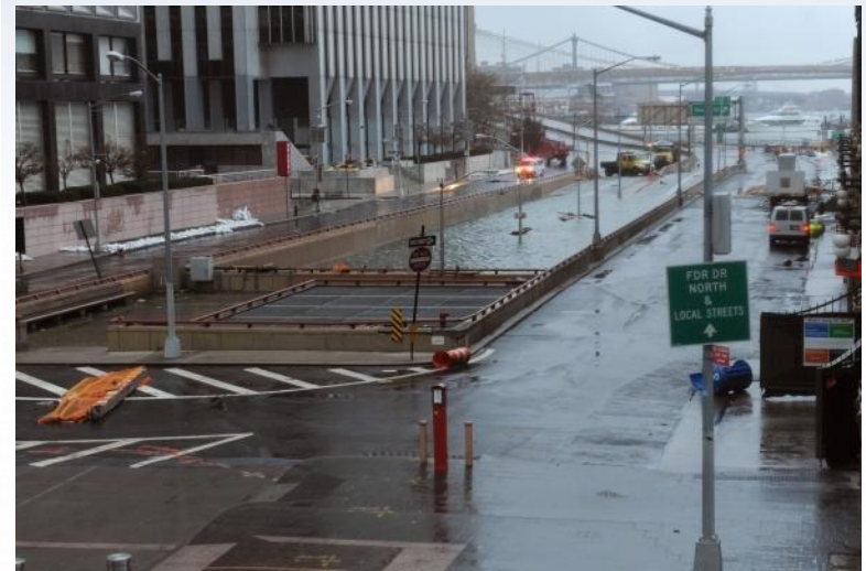
Battery Park underpass after Sandy hit
